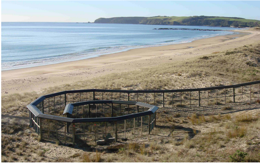
Figure 2. Photo showing the koru design at the end of the Tawharanui Open sanctuary predator fence; note the length of beach visible between fence end and the sea. Photo: Matt Maitland
